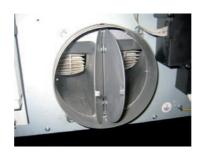
For hoods with outside air exhaust, fit a check valve to prevent wind and returning air from entering.
